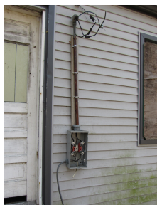
Exposed conductor
