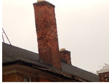
Open mortar joints
