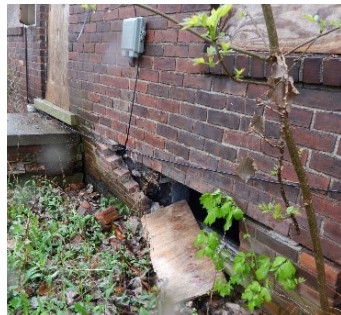
Failed exterior brick wall
