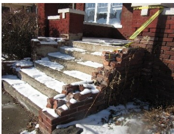
Collapsing porch wing wall
