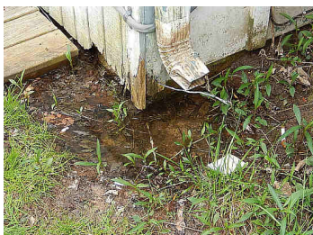
Pooling water near foundation
