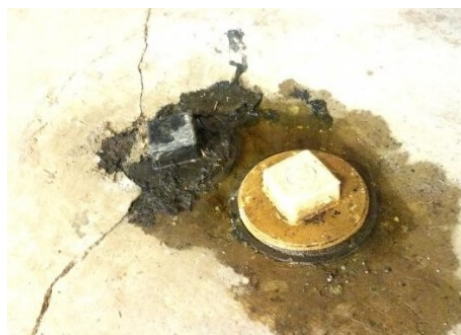
Leaking clean out plug
