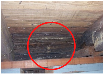
Rotted subflooring and joist
