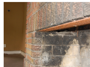
Damaged firebrick
