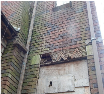
Missing brick above lintel
