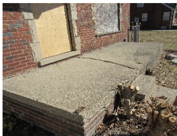
Cracked porch deck
