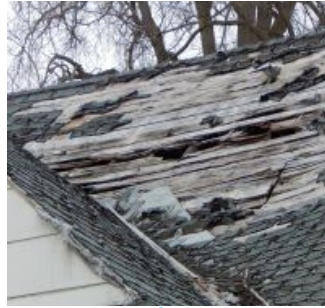
Exposed roof deck
