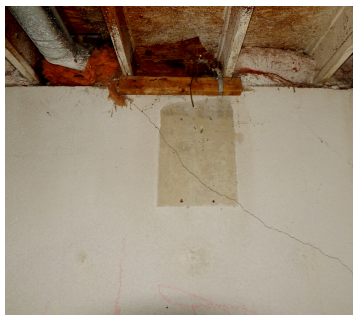
Cracked poured foundation
