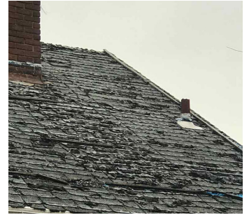
Deteriorated shingles
