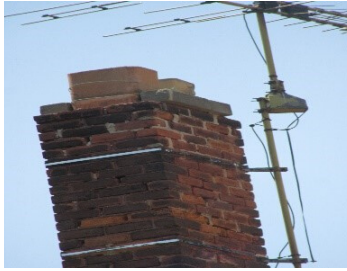
Missing chimney cap
