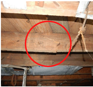
Cracked joist
