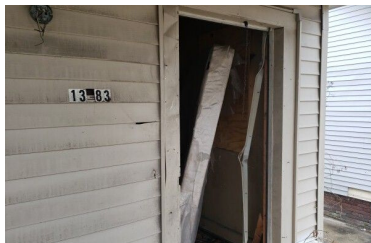
Missing door, damaged frame
