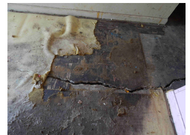
Cracked slab foundation
