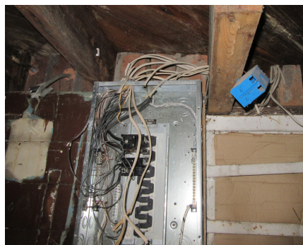
Cut and missing wiring
