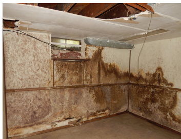
Evidence of water intrusion
