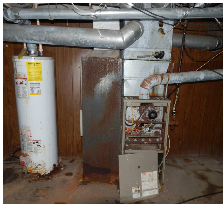
Water damaged furnace and water heater
