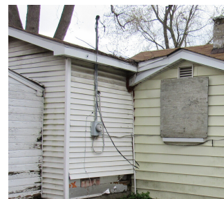
Exposed wires
